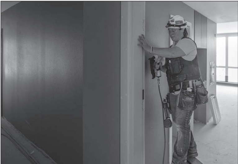
Apprentice carpenter Summer Smith, a member of Local 1503 and an RDF Builders employee, installs wood trim in a doorway.
